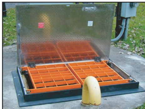
Closed Safety Grates Provide 300 P.S.F. pedestrian rated fall through protection
